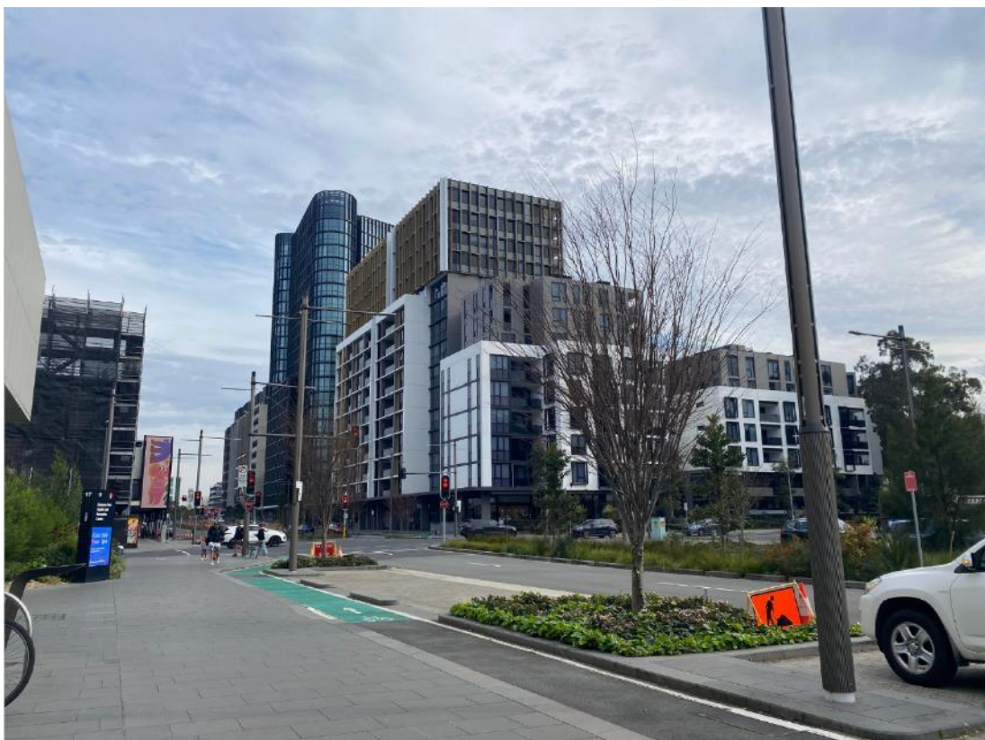
Figure 6: Looking west along Zetland Avenue
