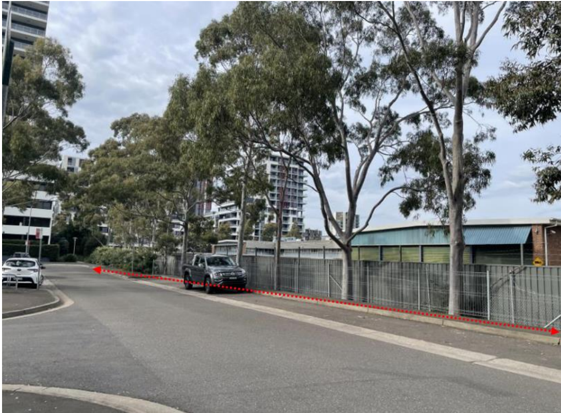
Figure 7: Site viewed from Kirby Walk
