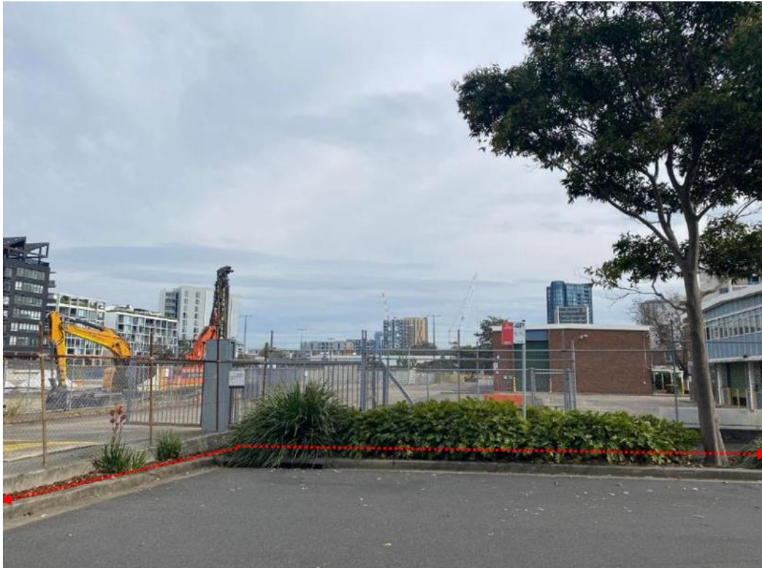
Figure 9: Site viewed from Defries Avenue looking west
