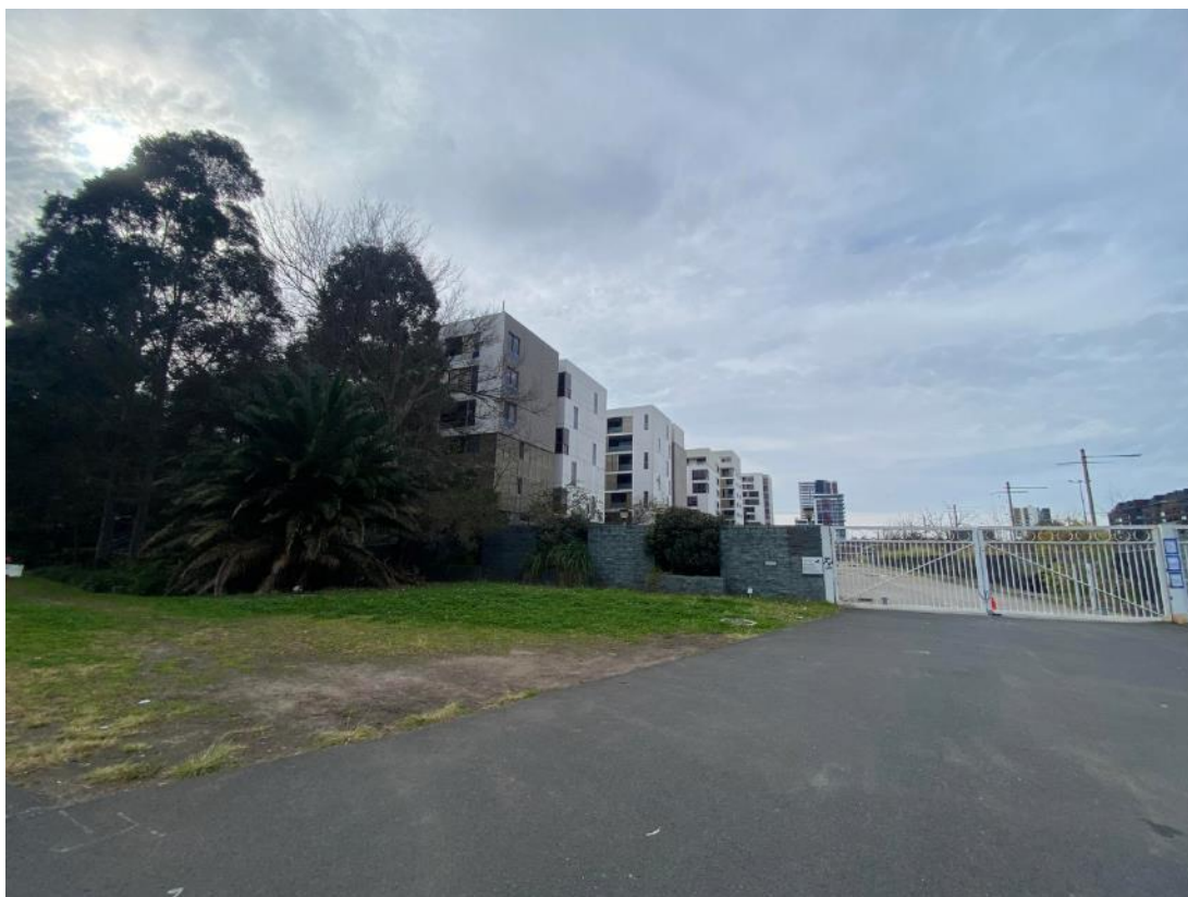
Figure 2: Site viewed from Joynton Avenue looking east
