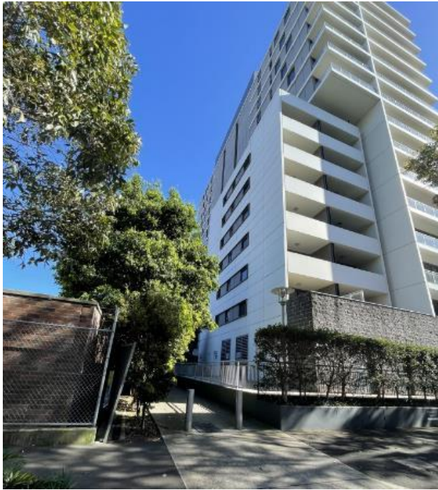
Figure 54: Southern facade of 8 Ascot Avenue, viewed from Defries Avenue looking west
